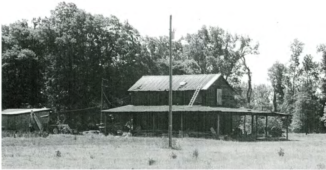
Figure 36. Property 7 - House and Outbuildings. Both views looking south. The property has been determined not eligible for the National Register because it is neither historically nor architecturally significant. Photographed May 24, 2001.
