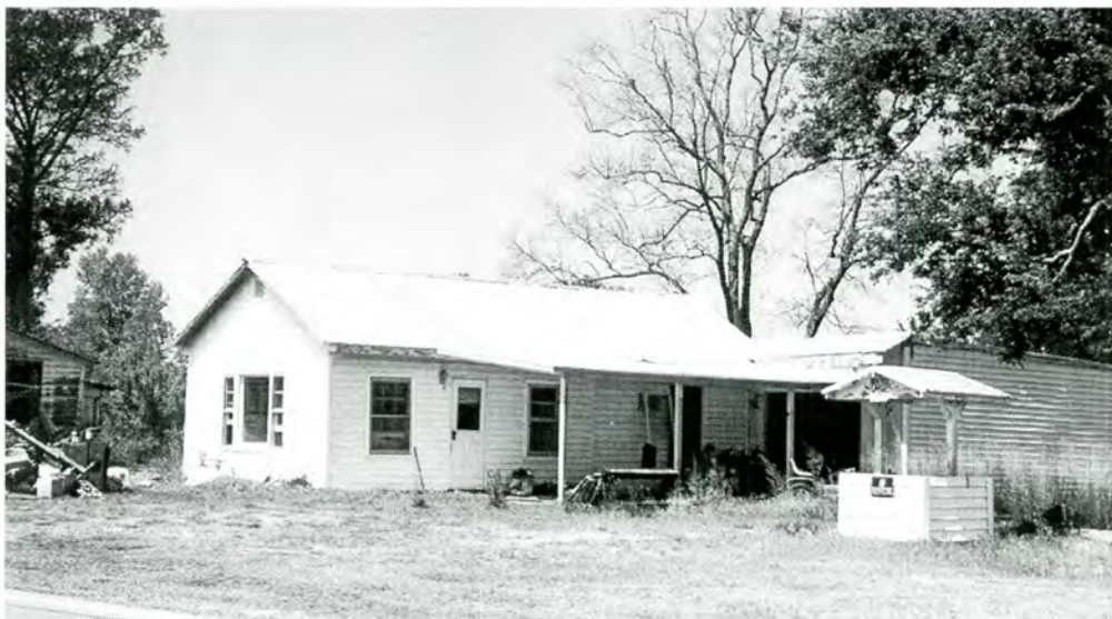
Figure 38. Property 9 - House. The property has been determined not eligible for the National Register because it is neither historically nor architecturally significant. Photographed April 26, 2001.
