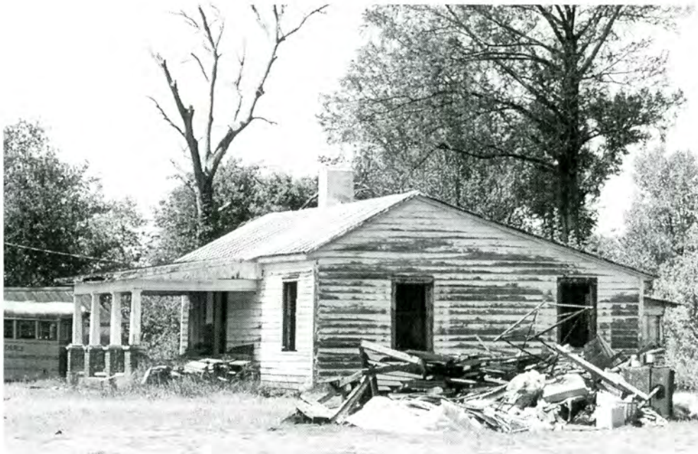
Figure 37. Property 8 - House. The property has been determined not eligible for the National Register because it is neither historically nor architecturally significant. Photographed April 26, 2001.
